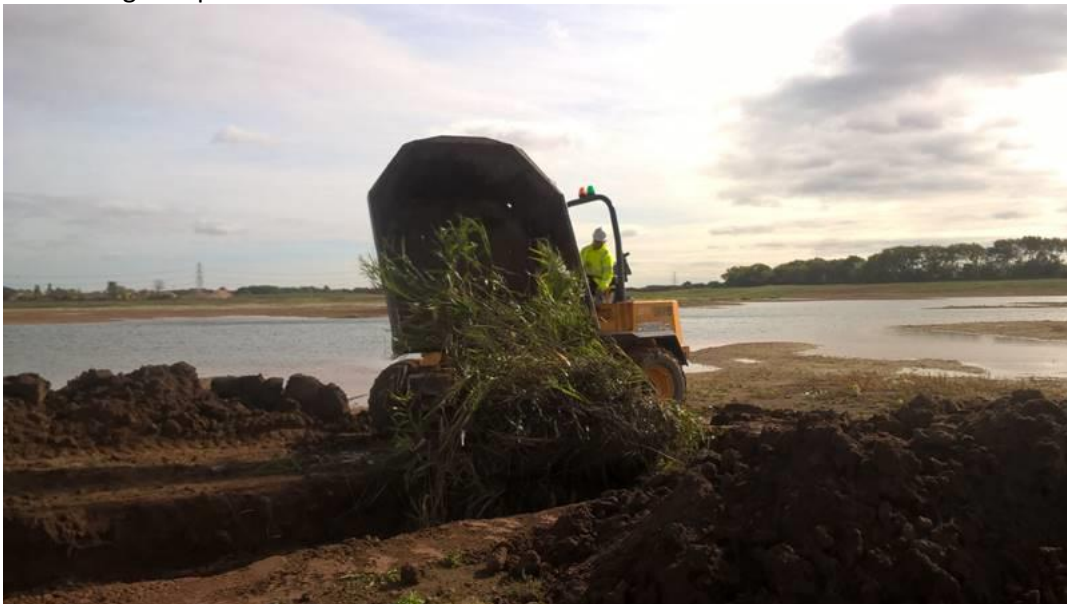
Reed being dumped into trench.
